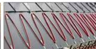
Construction heating systems based on heating cables
